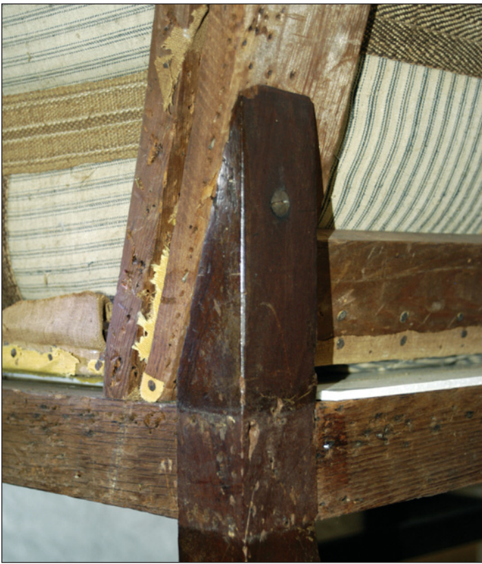
Fig 4: Evidence of “boxed” nailing. Image also shows tusk on rear leg. Photography by Steven Crossot. Courtesy of the Philadelphia Museum of Art.
